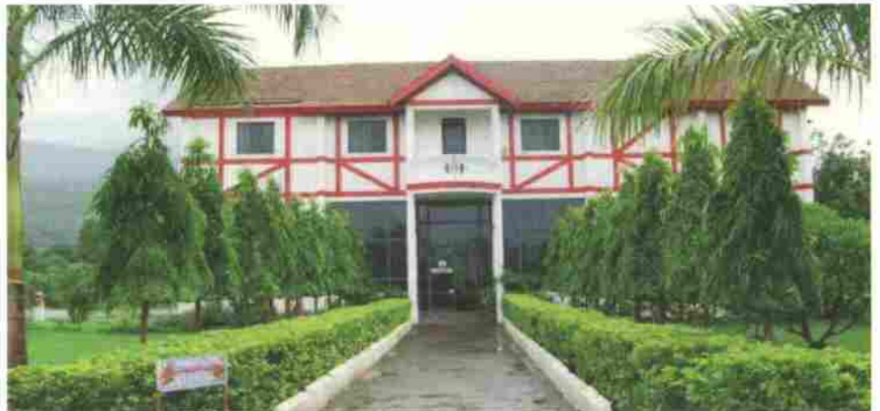
AE's training academy was rebuilt from a former school.
